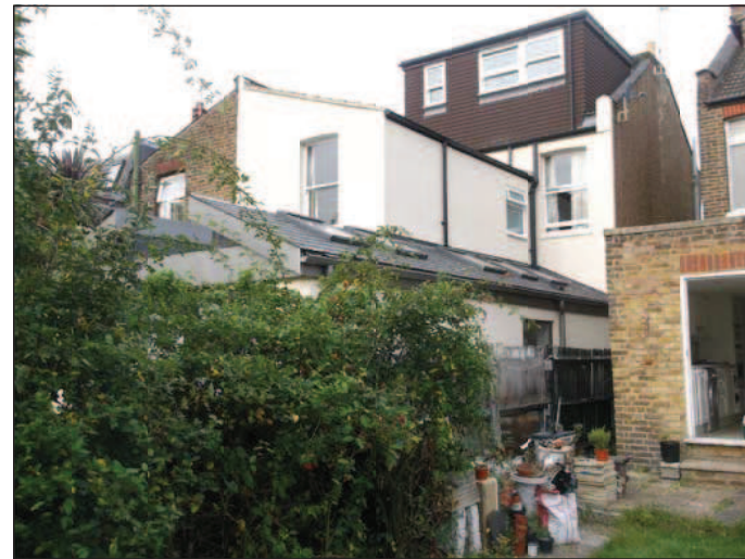
View of 26 Rayleigh Road's extension
