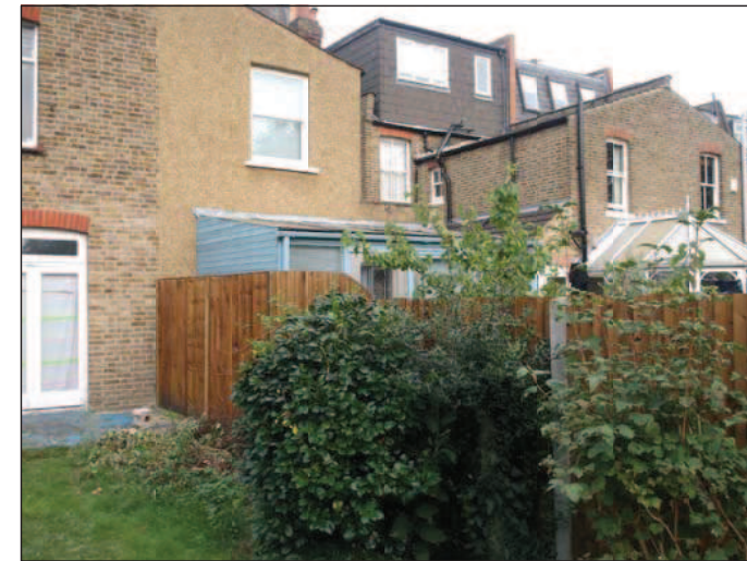
View of 22 Rayleigh Road's extension
